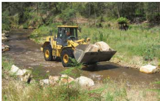
Boulders were placed in-stream according to a plan developed with North East CMA – June/Dec 2015.
